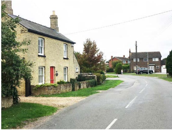
Figure 18 Mill Road looking west.
