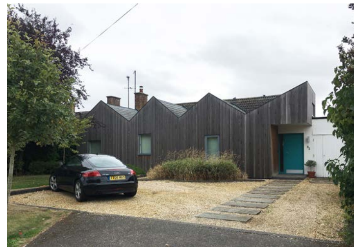
b: A characterful extension whose form is not typical of the houses in Over but which uses a single primary material sympathetic in tone to the existing pantile roof.
