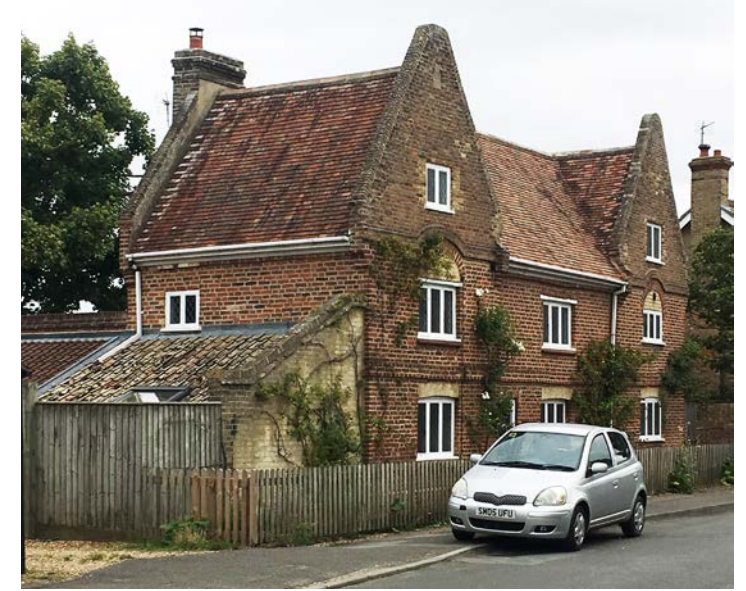
Figure 43: material integrity High Street: number 22. Consistent palette of red brick walls and red clay tiled roof, with 'Dutch' gables.
